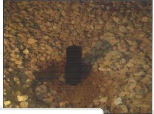
Figure 2 Pier is ready for head assembly
