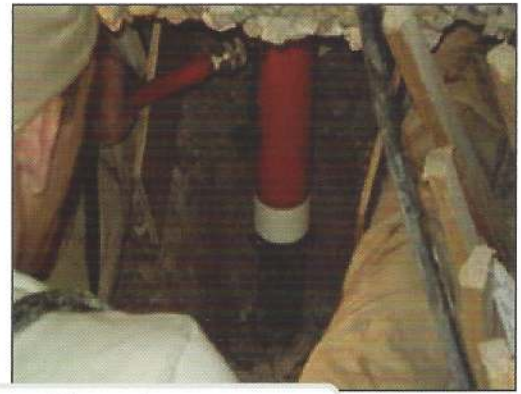
Figure 1 Pier is driven to bedrock under center of wall being lifted
