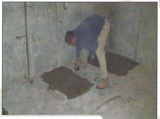
Figure 4 Immediate work area is filled in with new concrete
